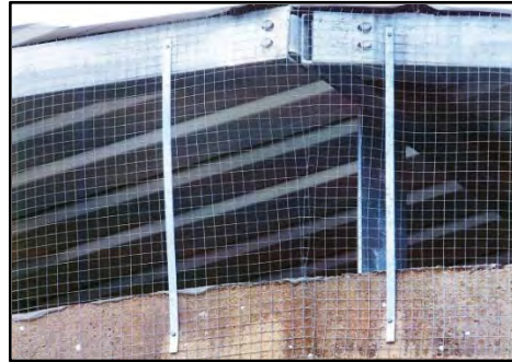
Photo 4 – Deficient reservoir roof design
