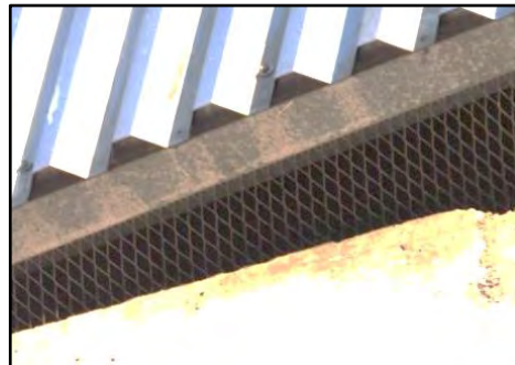
Photo 5 - Large mesh openings on reservoir
