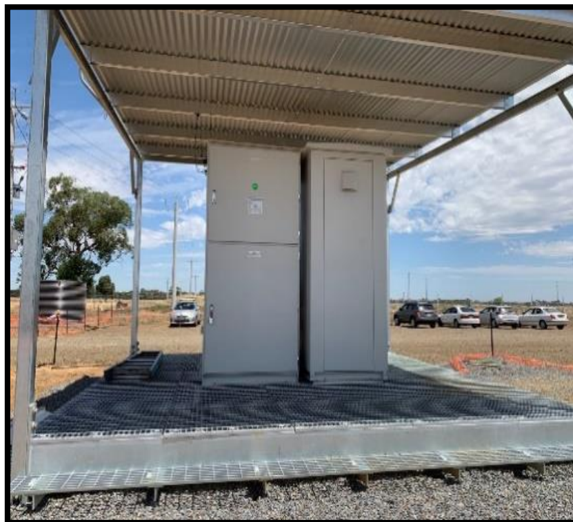
Figure 8 Typical HV switchboard and platform (Source: ACEnergy)
