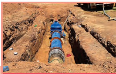
New Sewer Rising Mains (G2 to G1 Sewer Pump Stations)
