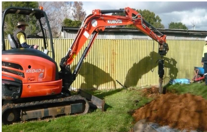
Excavating for the Tank
