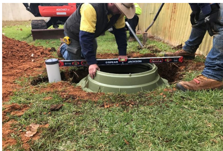
Placing the Tank
