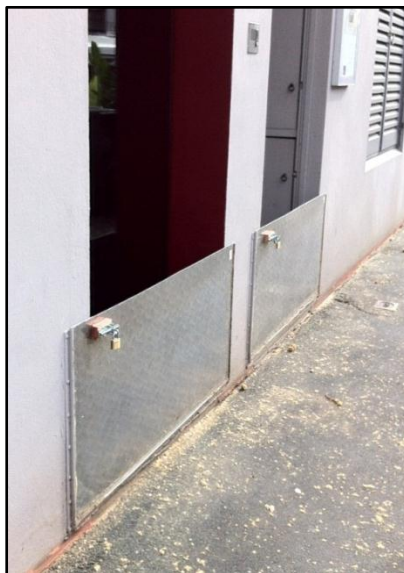
Photograph 3: Flood Gate at Front Door of Residential Property
