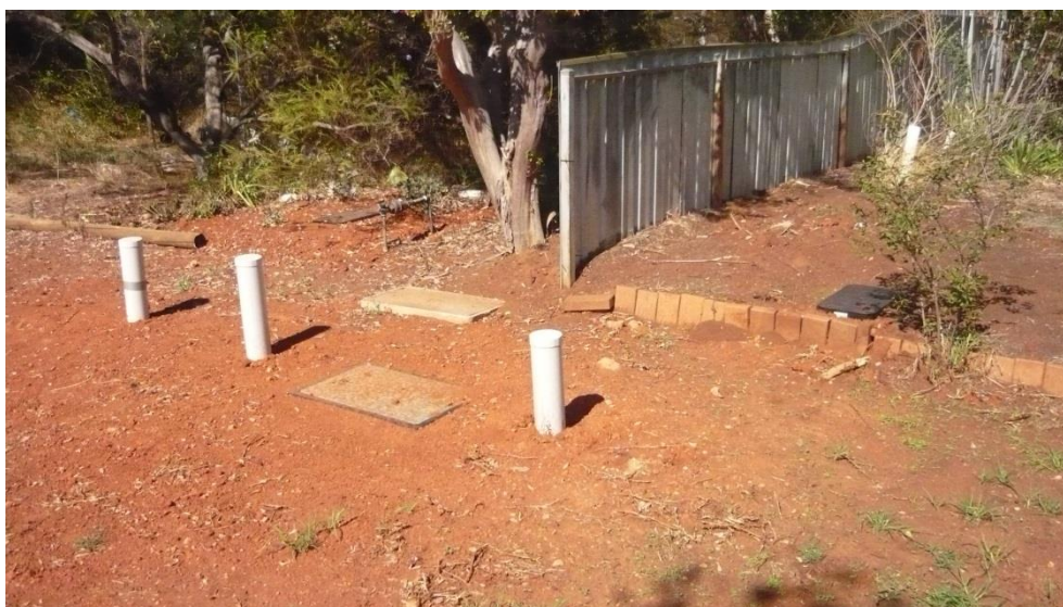
Partly completed flush point at Tharbogang
