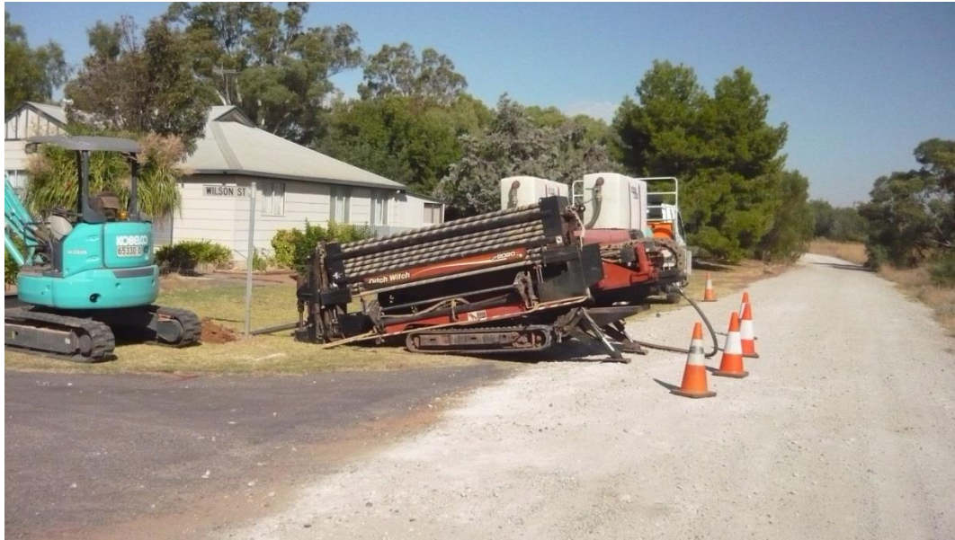
Directional boring works at Nericon
