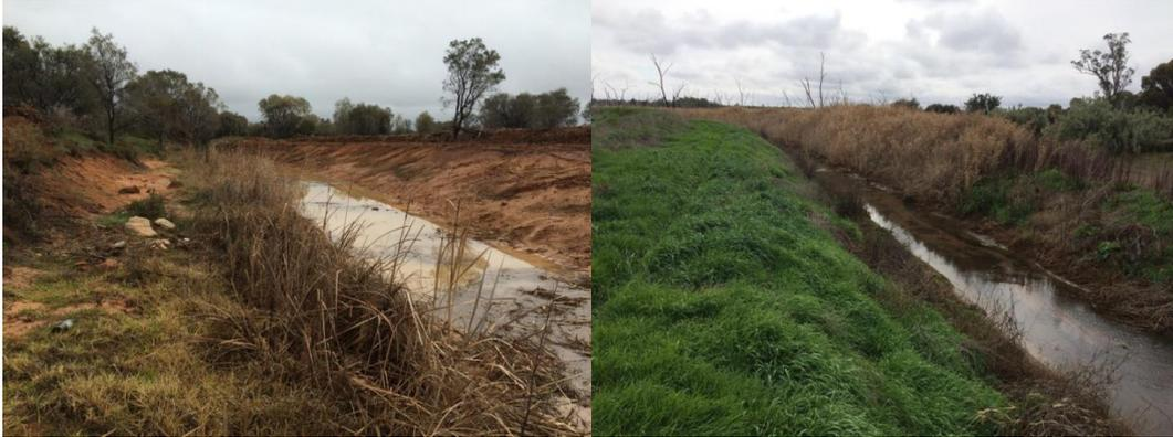
**Figure 3-30** Recent (left) and old (right) drain cleaning evident with Cumbungi and Common Reed retained on one bank
