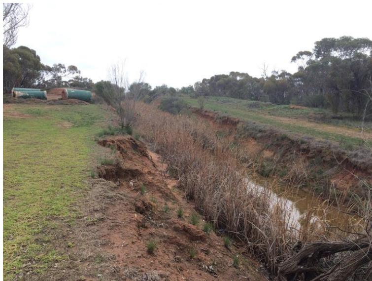
*Figure 3-28 Drain Canal showing terrestrial vegetation on the upper bank and aquatic vegetation in the bed*
