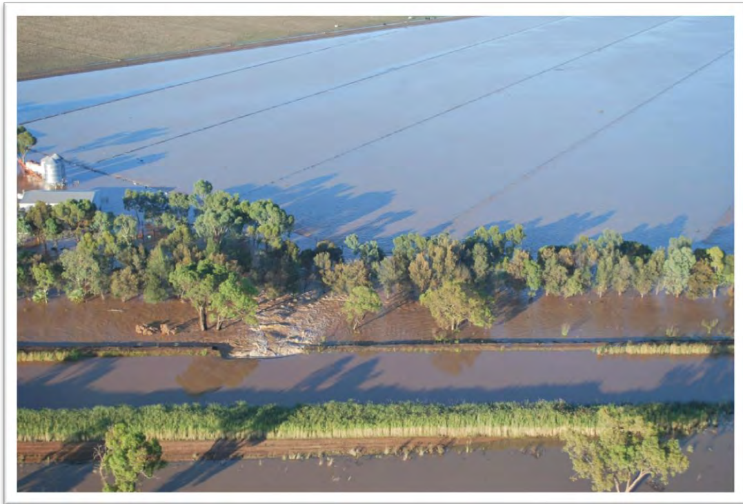
Figure 8-26 Main Canal Breach at Parizotto's during the March 2012 Flood Event
